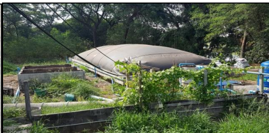
Figure 2 Plug Flow Digester
